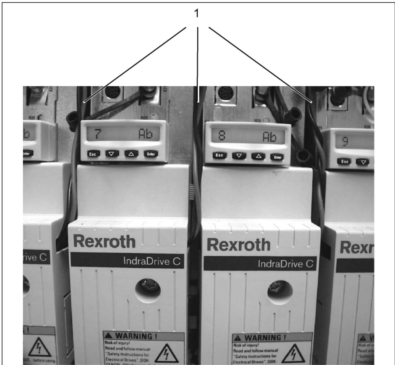
1: lines to control voltage supply
